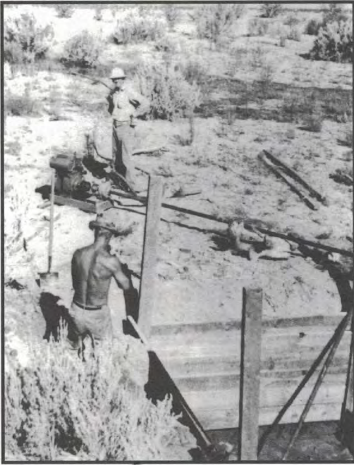
Above: Howard Kimmerle standing by the pump (center of photo). Man in foreground is probably John Kimmerle, who looks like he is tamping the dirt around the form.
