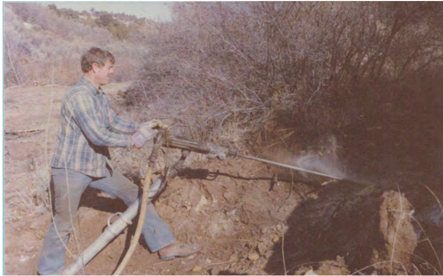
(Pictured: David Kimmerle starting a new mine portal.)
