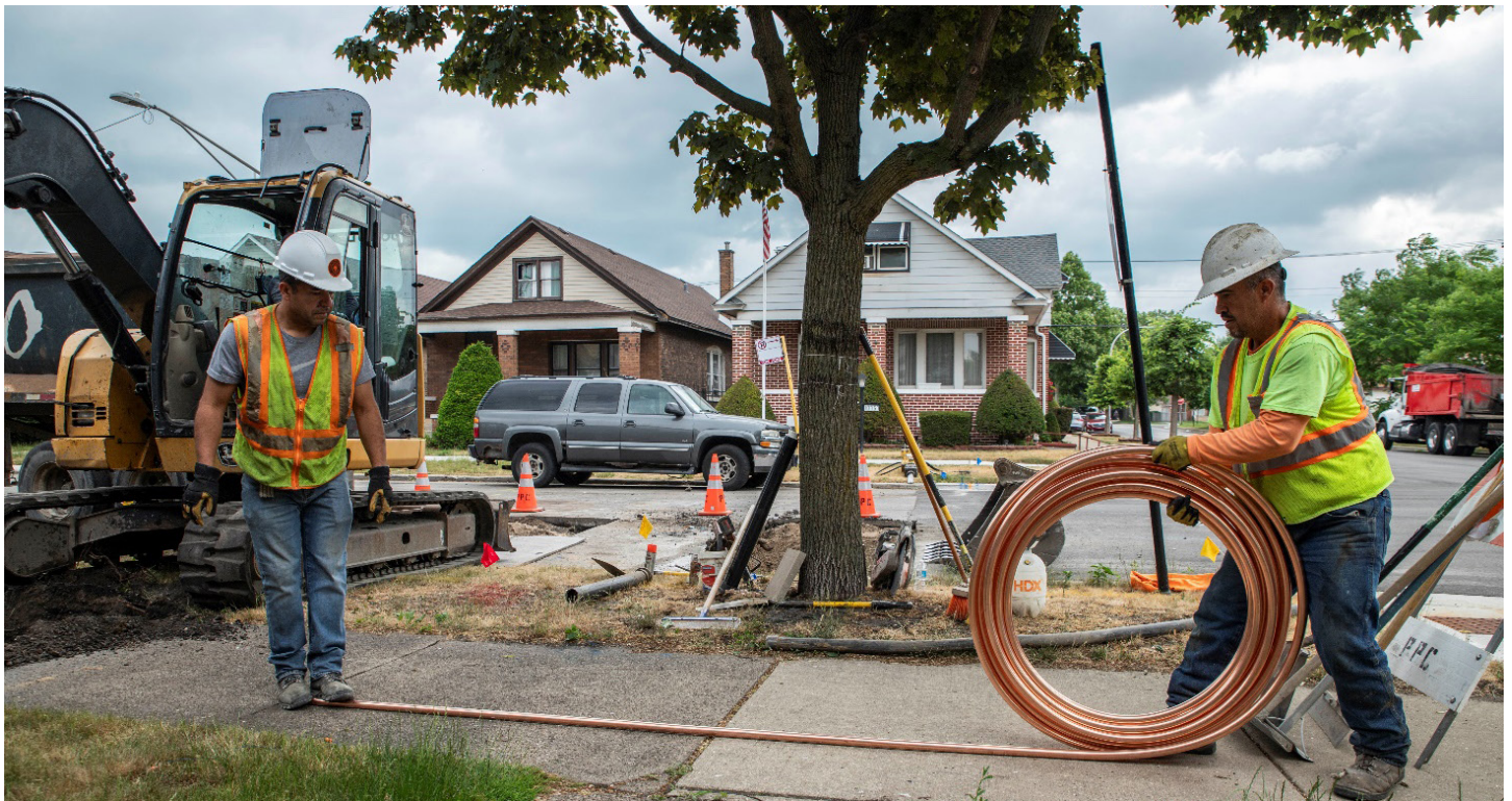
Workers unrolling new copper line outside a home in Chicago, Illinois.
