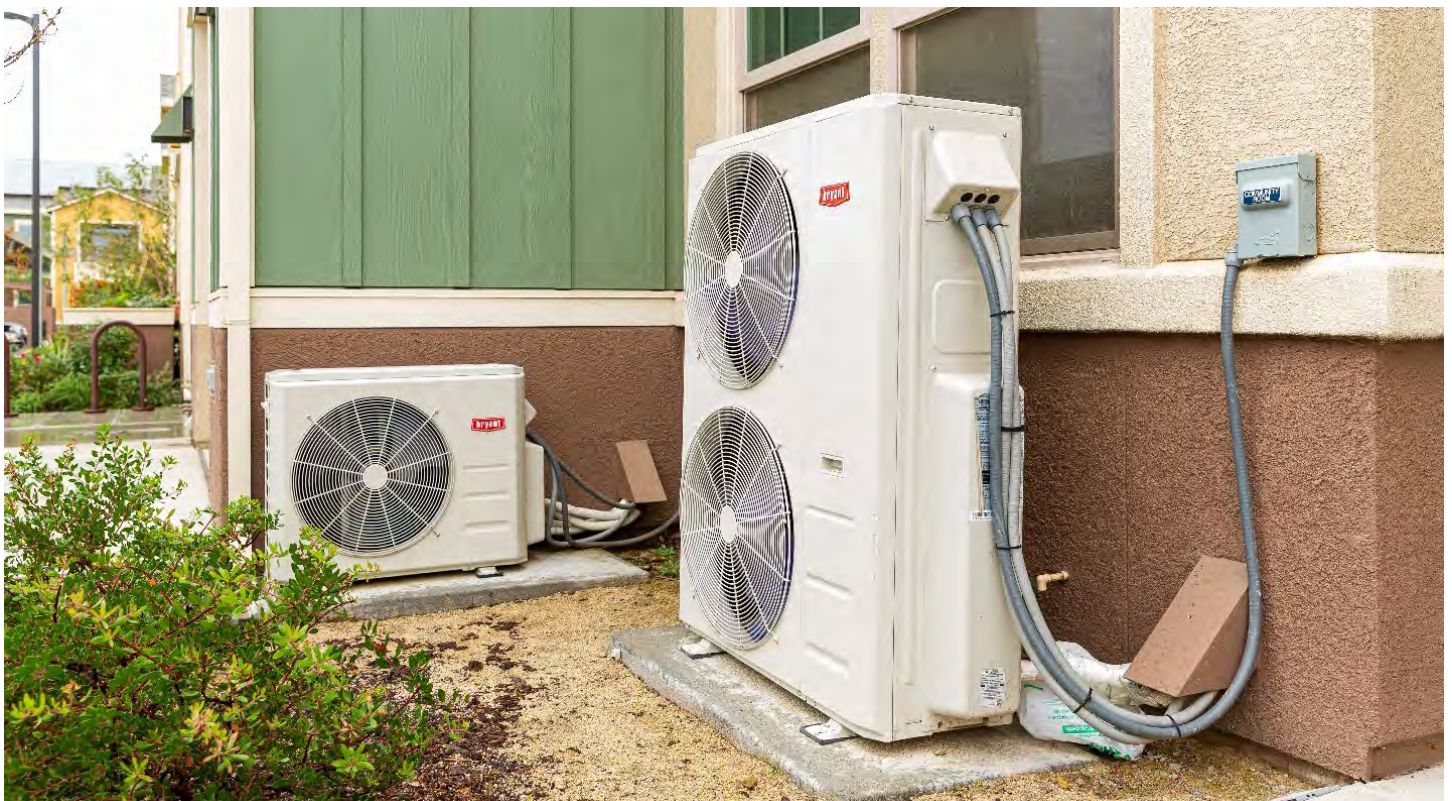
Heat pumps are all-electric and can provide both efficient heating and cooling.
