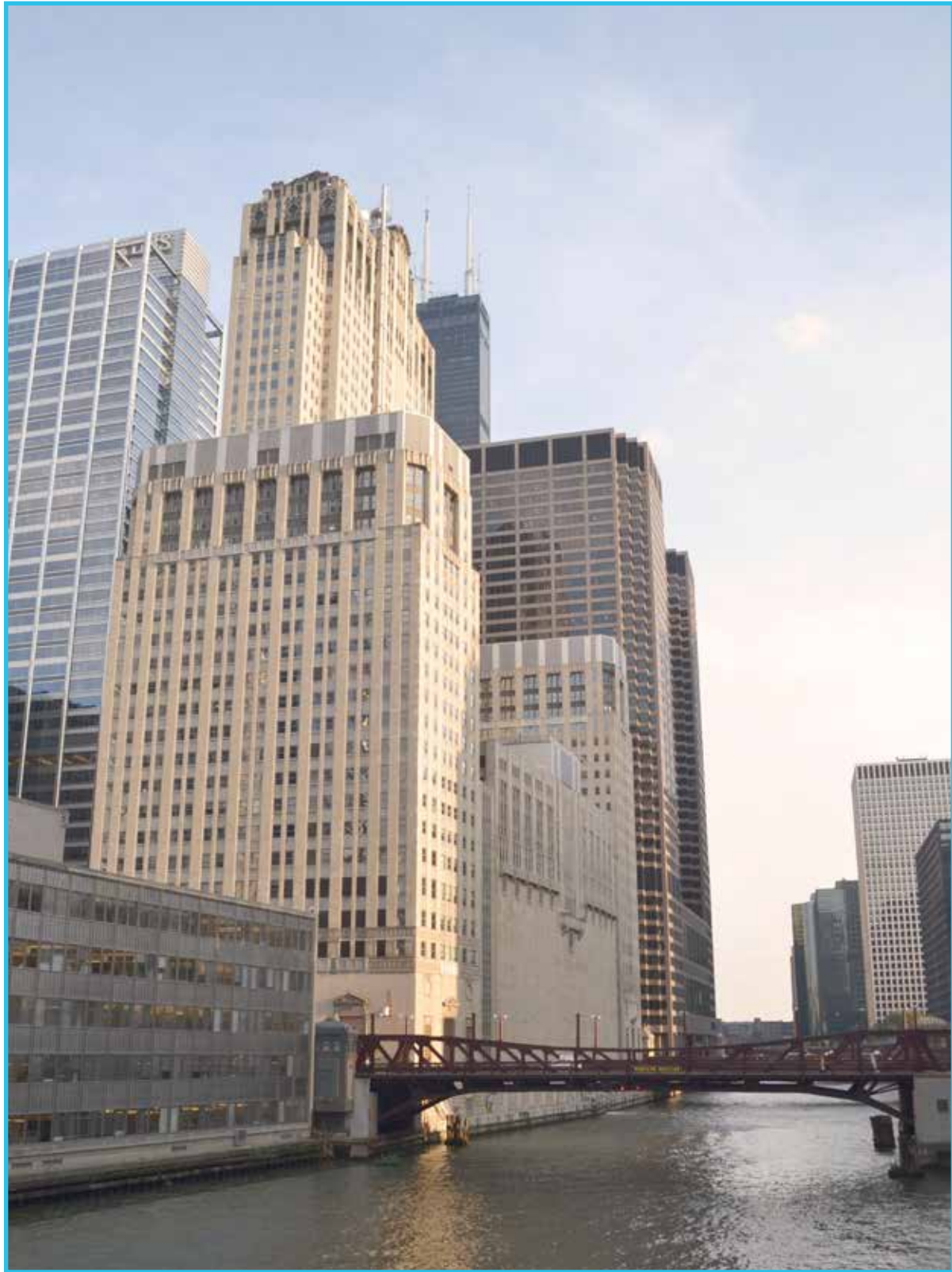
Clockwise from left to right: A) View of 20 N. Wacker. B) Stairs leading to the Washington/Wells CTA stop. C) Local Divvy bike-rental commuters. D) A woman commutes to work by walking. E) View within the Midwest office looking West.
