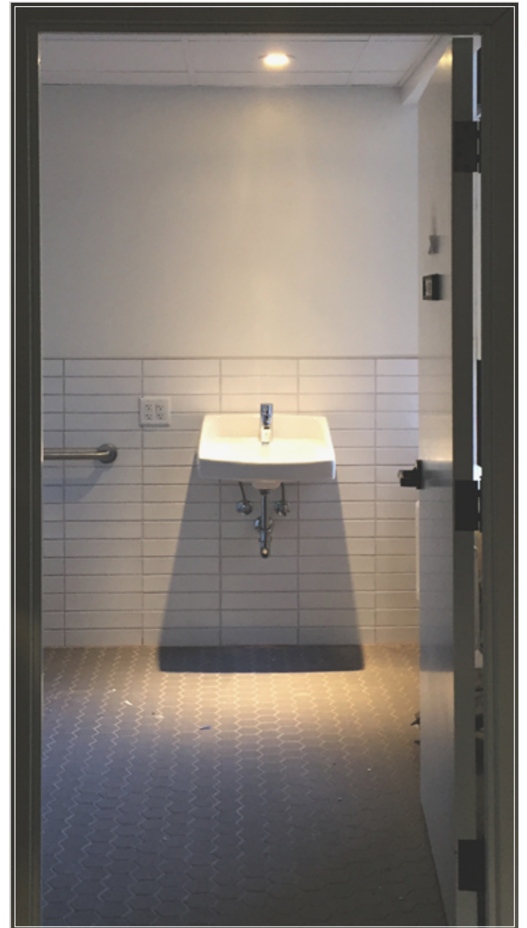
Sinks with aerators were installed to conserve water.
