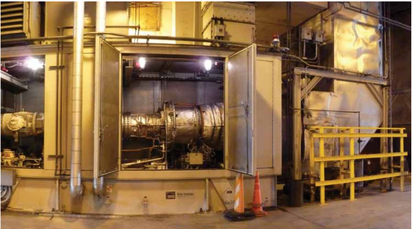
CHP system—gas turbine (center), with hot gases heading to heat recovery steam generator (right).
