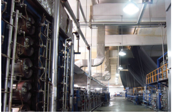
Better Insulation of steam pipes and valves
